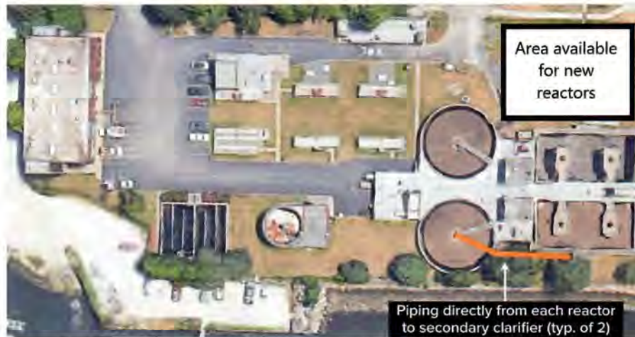
Figure 3. WWTF prior to upgrade
